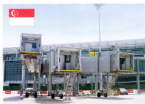
Changi International Airport (Singapore)
