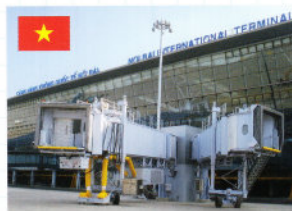
Noi Bai International Airport T2 (Vietnam)
